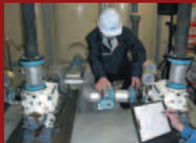
Plumbing and sanitation installation work
