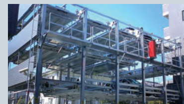
Metal members of a multilevel car parking tower
